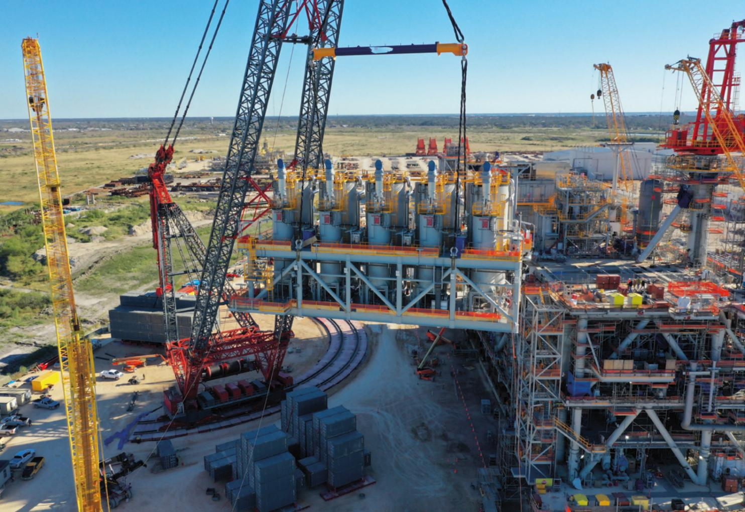
**The higher the crane capacity, the lower the number of modules needed**
