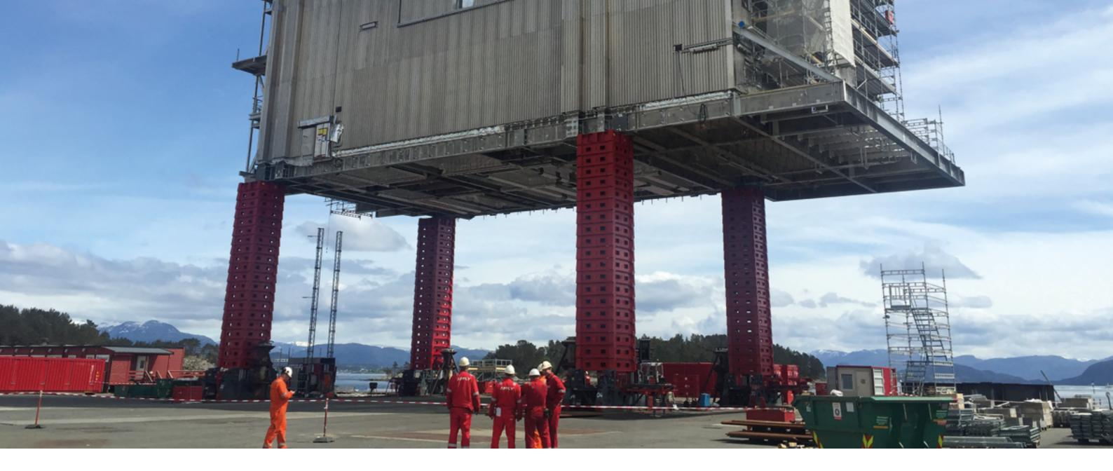
The Mega Jack 800 bridges the gap in jacking capacities between conventional 60t - 500t climbing jack systems and the Mega Jack 5200. This allows it to offer the same core efficiency and safety benefits of the larger system, but for a different, complementary range of project sizes and scopes.
