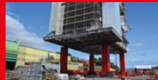
JACK-UP AND MATING OF MODULES, NORWAY
