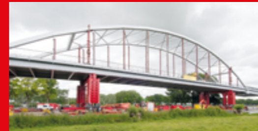
EXCHANGE OF THE LOENERSLOOTSE BRIDGE OVER THE AMSTERDAM-RIJN CANAL, THE NETHERLANDS
