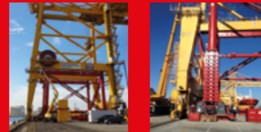
JACKING OF THREE STS CRANES, SPAIN
