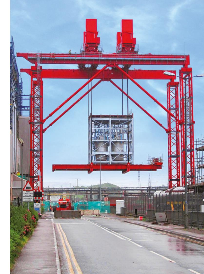
A simple gantry is assembled from a combination of two or more towers and an overhead beam or girder construction.
