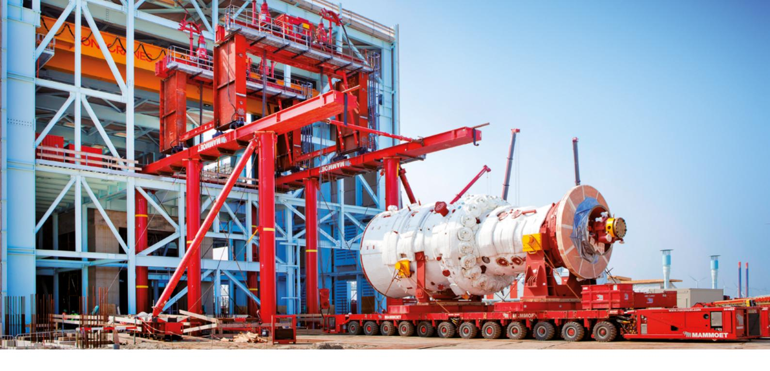
Mammoet Gantries can lift extremely heavy loads and are particularly well-suited in situations where only a small work area is available. This makes them an ideal and cost-effective choice for loads that exceed the capacity of the strongest crane, and for projects in the narrow confines of plants, factories and refineries.
